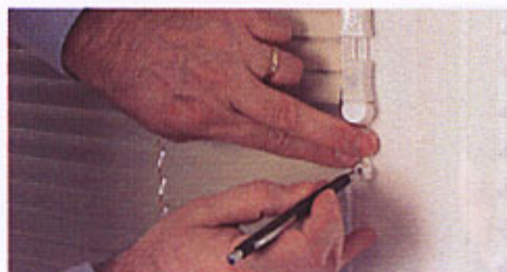
b2. Remove pulley cover, lightly tension lift cords down window side, mark position to fix pulley
