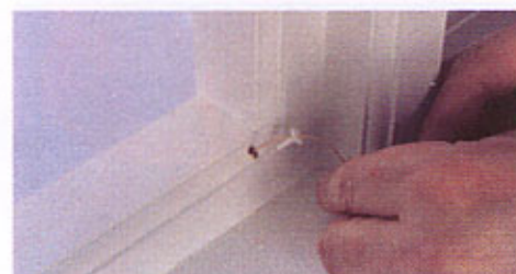
a4. Push cord knot into brass insert, push grommet into brass insert, aligning groove to cord
