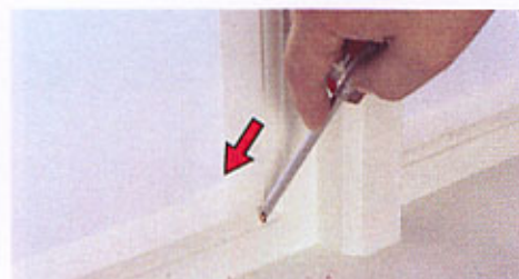
a3. Screw in brass inserts until flush with timber surface
