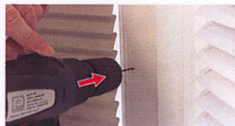
b3. Drill Ø2.5mm hole 1 off
